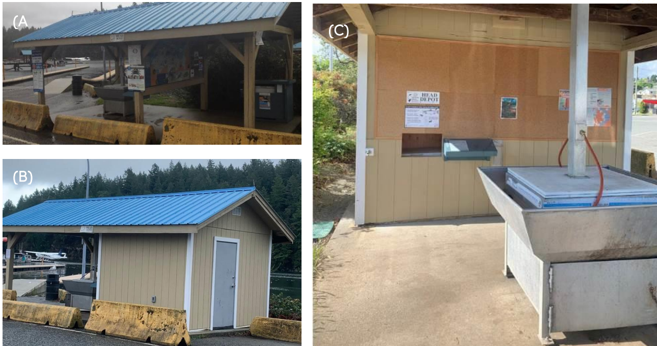
Figure 35. Images of the landing site at Brechin Marina before (A) and after (B and C) infrastructure upgrades conducted in July 2021 (photos by Kevin Pellett).
